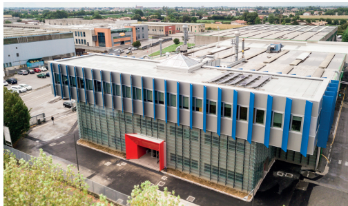
The Technology Centre in Cittadella (Padova) hosts technical and administrative facilities totally dedicated to research and development, designed and organized as a showroom where the world of Sirmax is shown live
